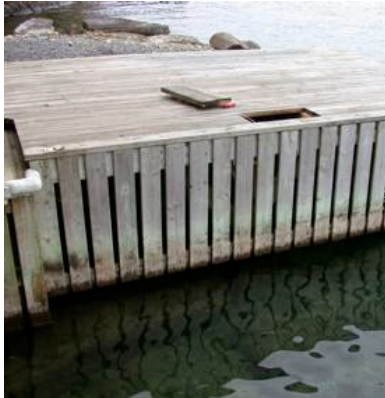
Figure 2a Water measurement column located under dock.
